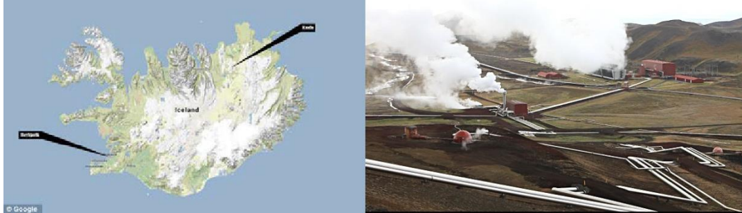
Krafla geothermal power station
